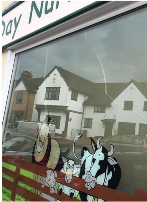
Photo of two cracks present in the outside face of a double-glazed unit. Vinyl graphics applied to the lower part of a window.
